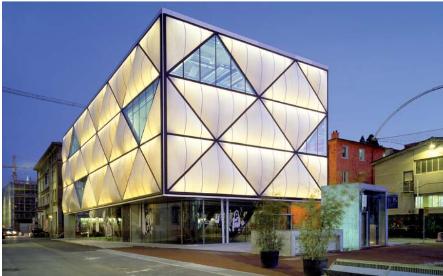
Abb. 5: La Miroiterie, Lausanne (Arch. B+W)
